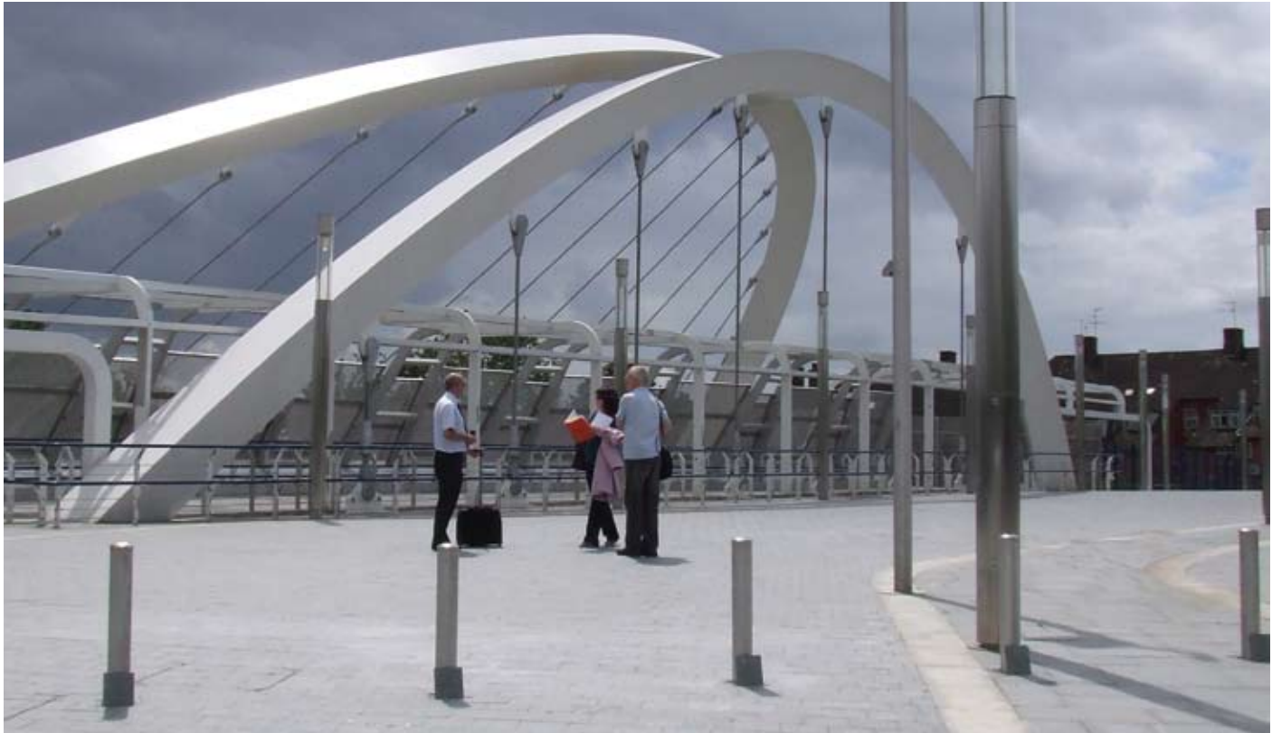
RT SS5 telescopic bollards, Wembley Stadium Station
