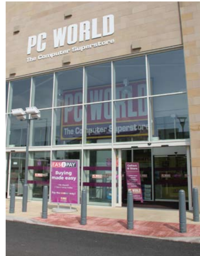
Ferrocast Anti Ram Bollards, PC World, Lancaster
